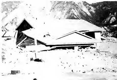
Photo 5. Collapsed dwelling in course of construction on Tucker Street near Pacoima Dam.
